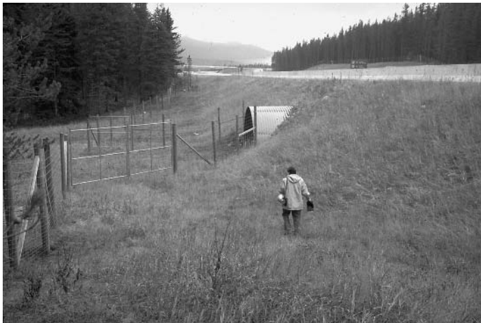
Fig. 7.1. Monitoring of mortality from vehicle collisions revealed severe impact on the large mammal populations of the Bow Valley in Banff National Park. Aggressive and expensive actions were taken to reduce this impact. The highway was fenced and large underpasses constructed to allow wildlife movement under the road. When it was discovered that some predators, most specifically wolves, would not use the tunnels, a large overpass was constructed. Wildlife underpass and roadside fence in Banff National Park, Canada. (Photographed by Paul F.J. Eagles.)
