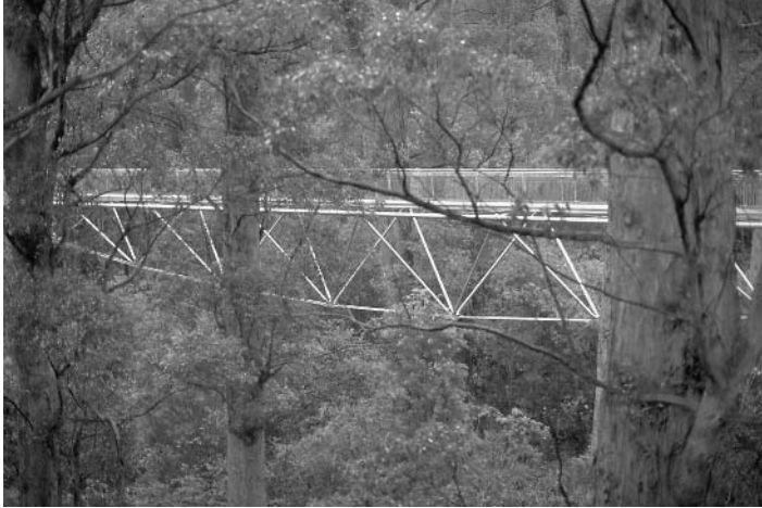
Fig. 8.5. The design and operation of park tourism services is a unique field. Specialized facilities provide exceptional visitor experiences. This highly engineered, but sensitively designed, treetop walkway allows visitors to experience the forest canopy of the giant red tingle trees of southwestern Australia. Treetop walk in Valley of the Giants, Walpole-Nornalup National Park, Western Australia. (Photographed by Paul F.J. Eagles.)
