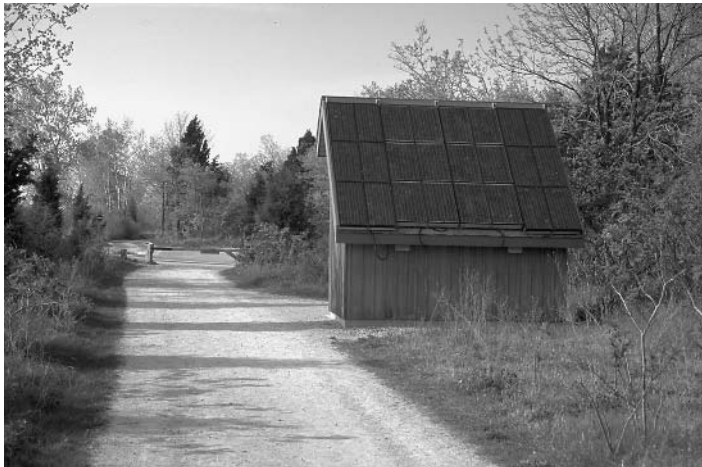
Fig. 8.2. The use of renewable energy sources is desirable in many park situations. This solar energy station in Point Pelee National Park provides power to a remote area of the national park. The station also provides interpretation information for the instruction of the visitor about the potential of solar electricity generation. Solar energy generation station in Point Pelee National Park, Canada. (Photographed by Paul F.J. Eagles.)
